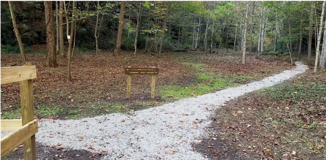
Photo: Recently completed Wildwood Trailhead
